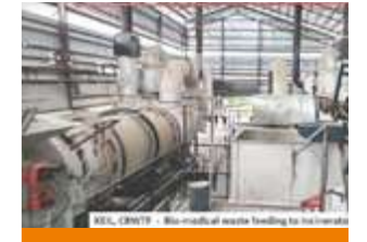
Bio-medical waste treatment facility
